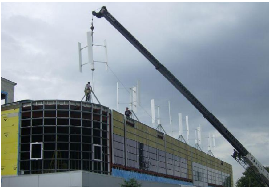
Figure 8 Installation of Roof Top Small Unit Vertical Axis Wind Turbine
